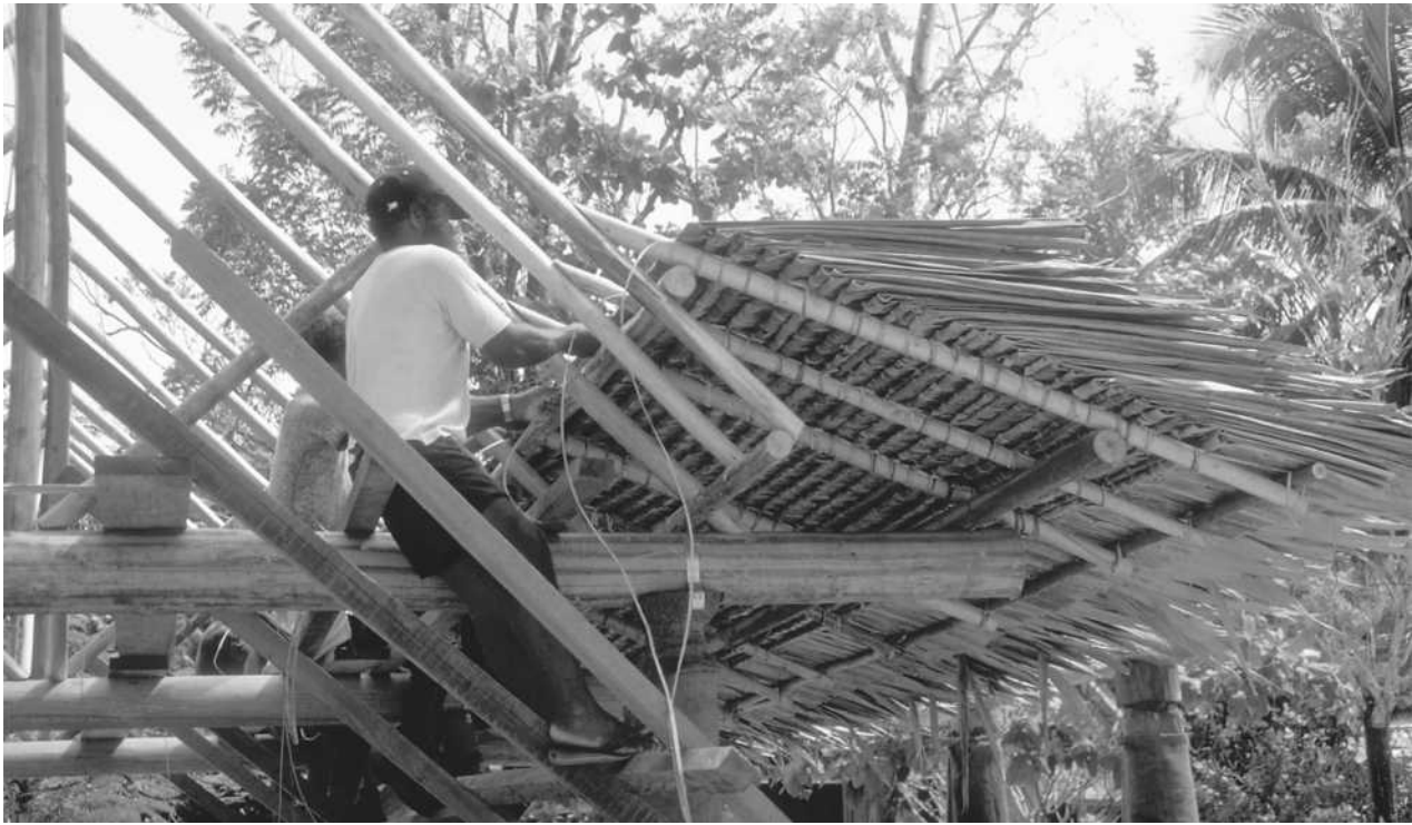
Workers tying thatch onto a new house in Honiara, Guadalcanal.
